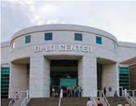
The Bi-Lo Center is an events center and entertainment destination serving the entire Greenville region. Source: Downtown Greenville Master Plan 2008
