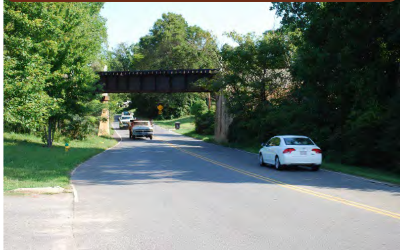
Rail Crossing at Salisbury Road
